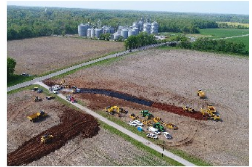
Beginning to break ground in Guthrie, Kentucky
