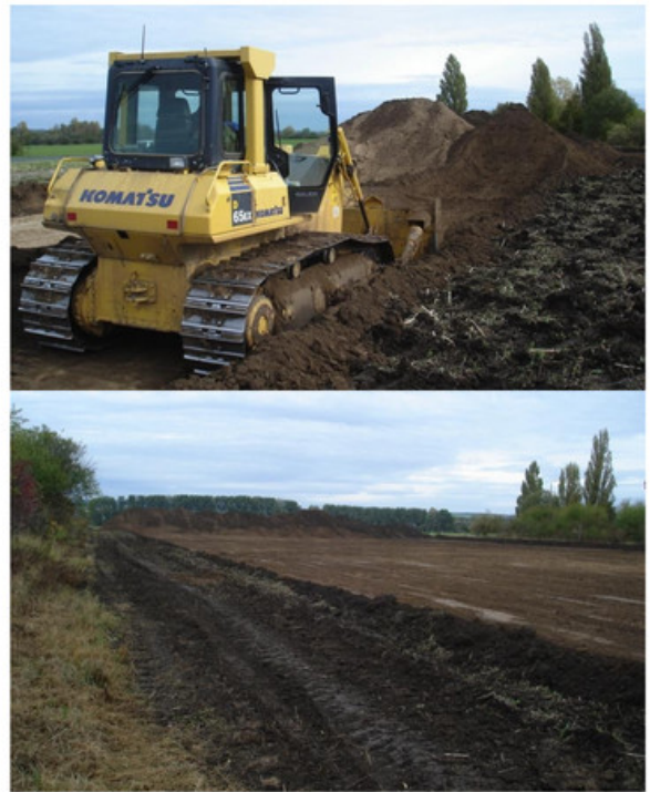
Broke Ground in Europe
