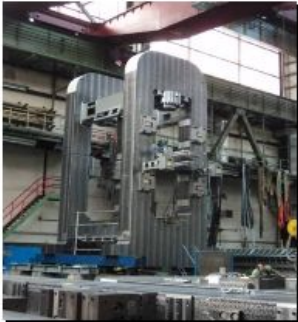
Pre-assembling Cold Mill stands
