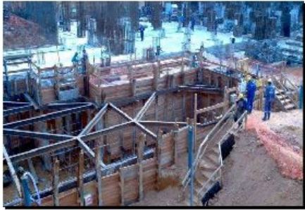
Line-D Casting Center Foundation
