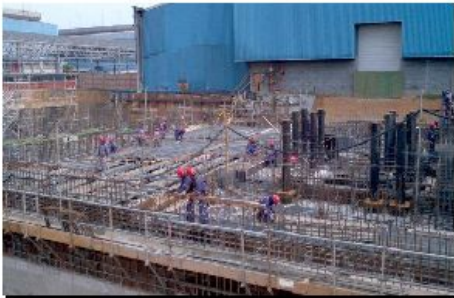
Cold Mill 3 Foundation
